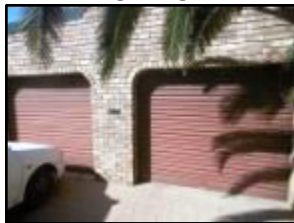
Out buildings: Double garage.
